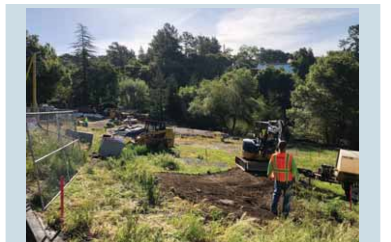
Work begins at MOFD Fire Station 43.
